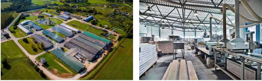
Figure 8. Factory site and aspiration systems
